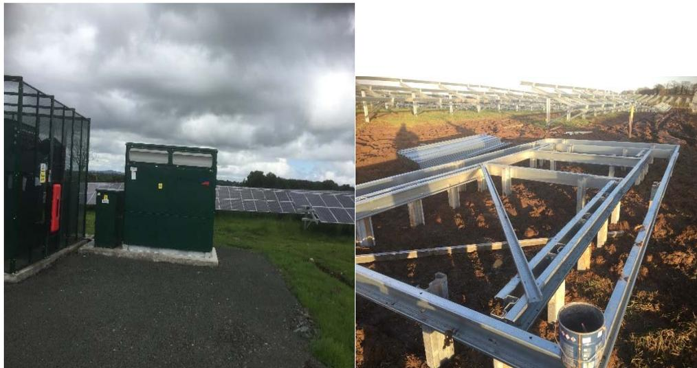
**Figure 2.3 Rock fill with concrete plinth foundation and Piled alternative**
