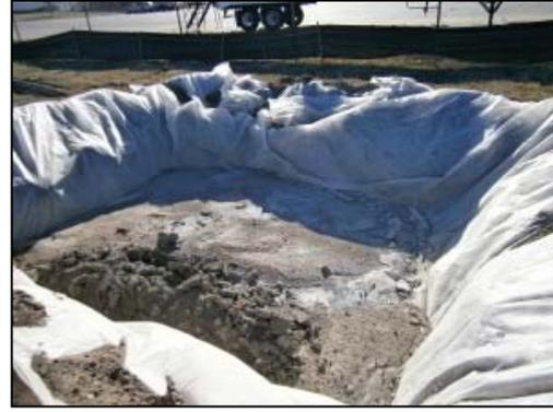
Plate 3.2 Concrete washout area
