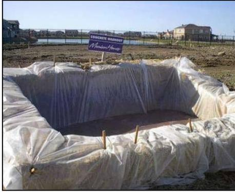
Plate 3.1 Concrete washout area
